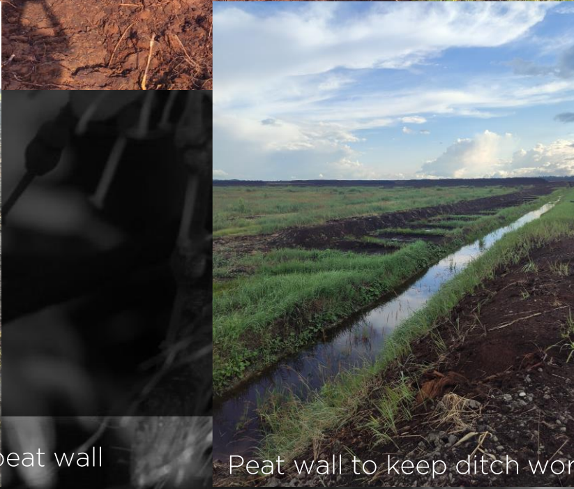
Complete closure of collector ditch
